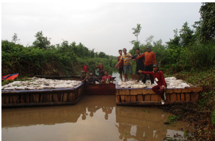
Figure 5 Construction of canal blocks
